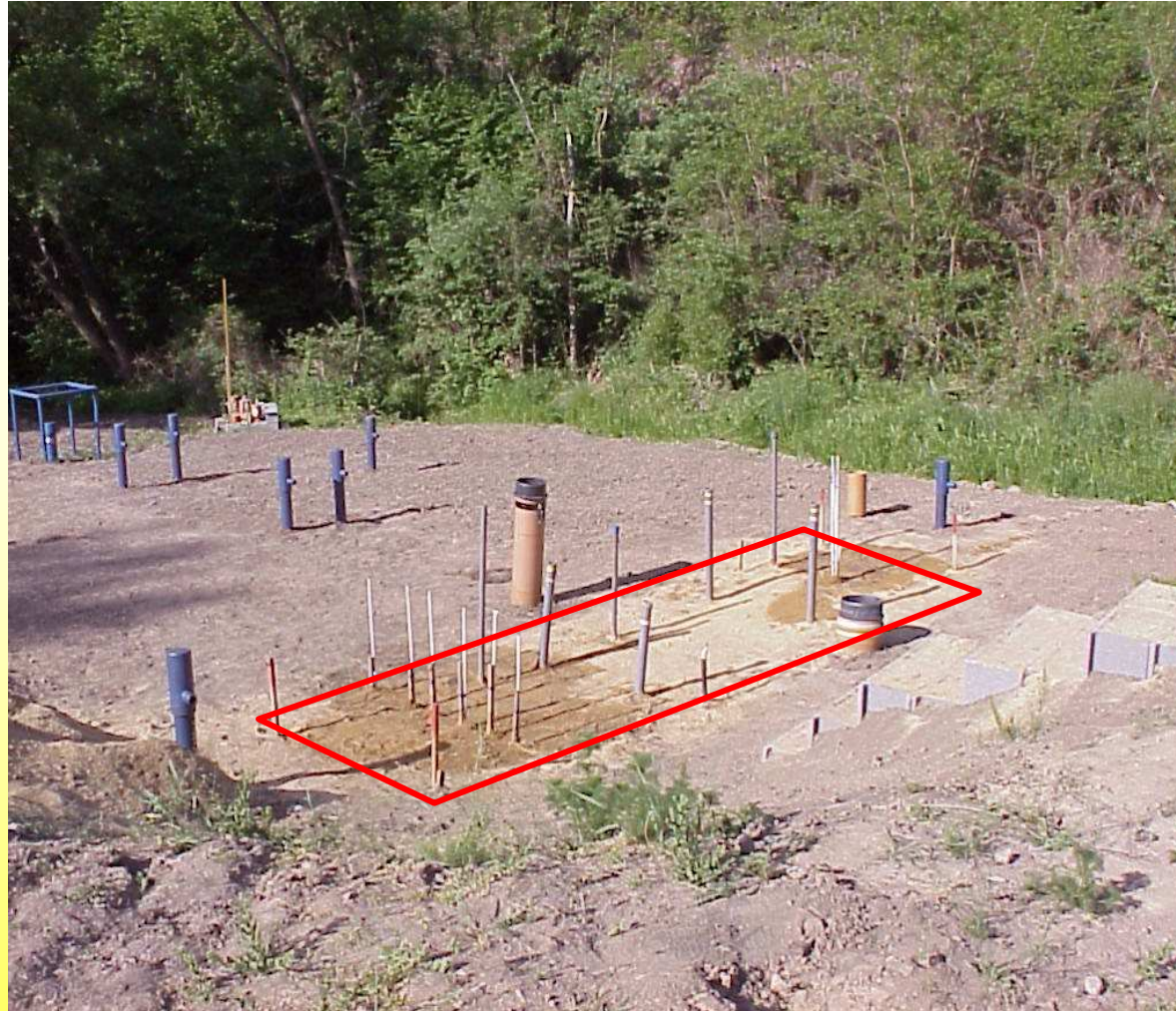
View of the experimental permeable reactive barrier with monitoring wells (Csővári et al.)
